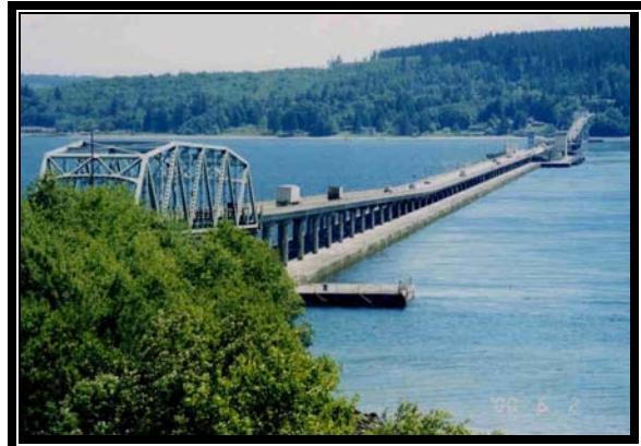
Fig. 3 Hood Canal Floating Bridge, USA
