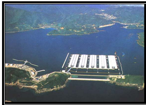
Fig. 10 Kamigoto Floating Oil Storage Base, Nagasaki Prefecture, Japan
