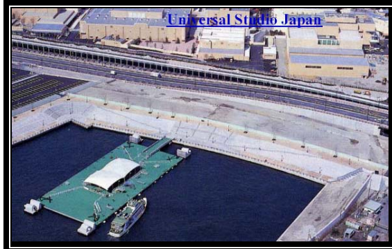
Fig. 12 Emergency Rescue Base in Osaka Bay
