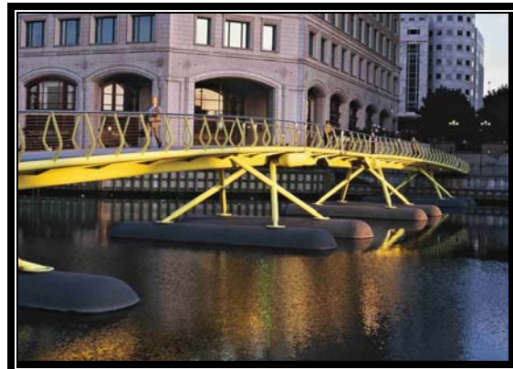
Fig. 5 West India Quay Footbridge, United Kingdom
