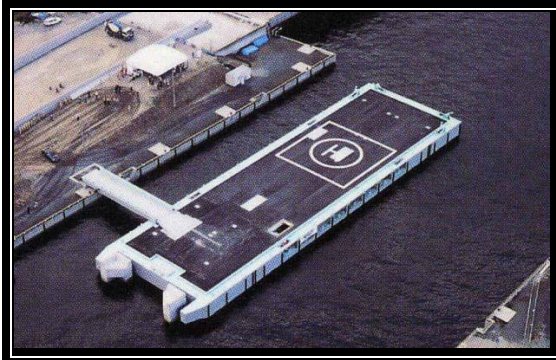
Fig. 11 Emergency Rescue Base In Tokyo Bay
